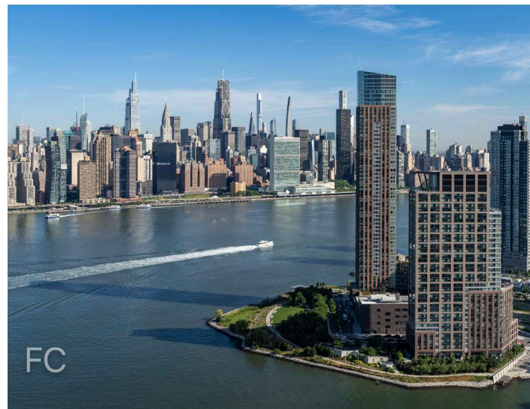
View to the northwest towards Midtown Manhattan and Hunters Point South.
