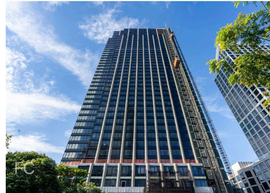
Looking up at the north facade.
