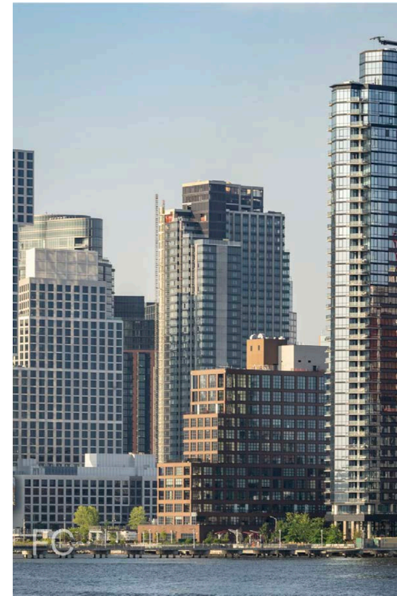
Southwest corner of the tower.
