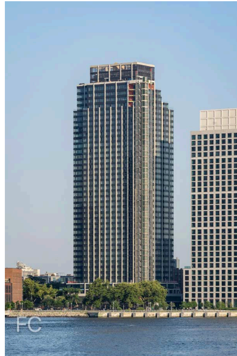
Northwest corner of the tower.
