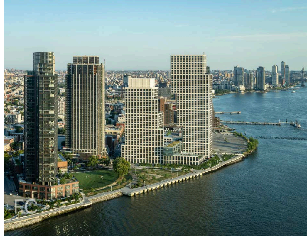
Two Blue Slip (left), 16 Dupont (center), and Eagle + West (right).
