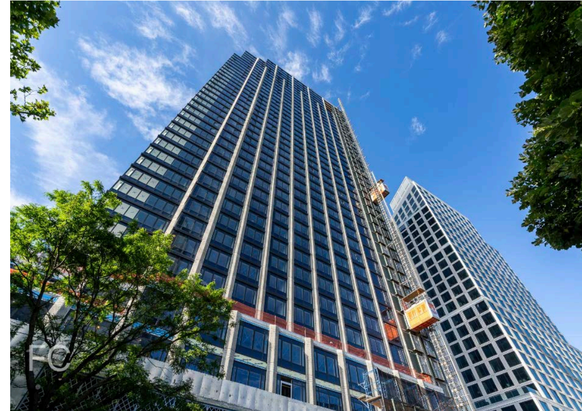
Looking up at the north facade.
